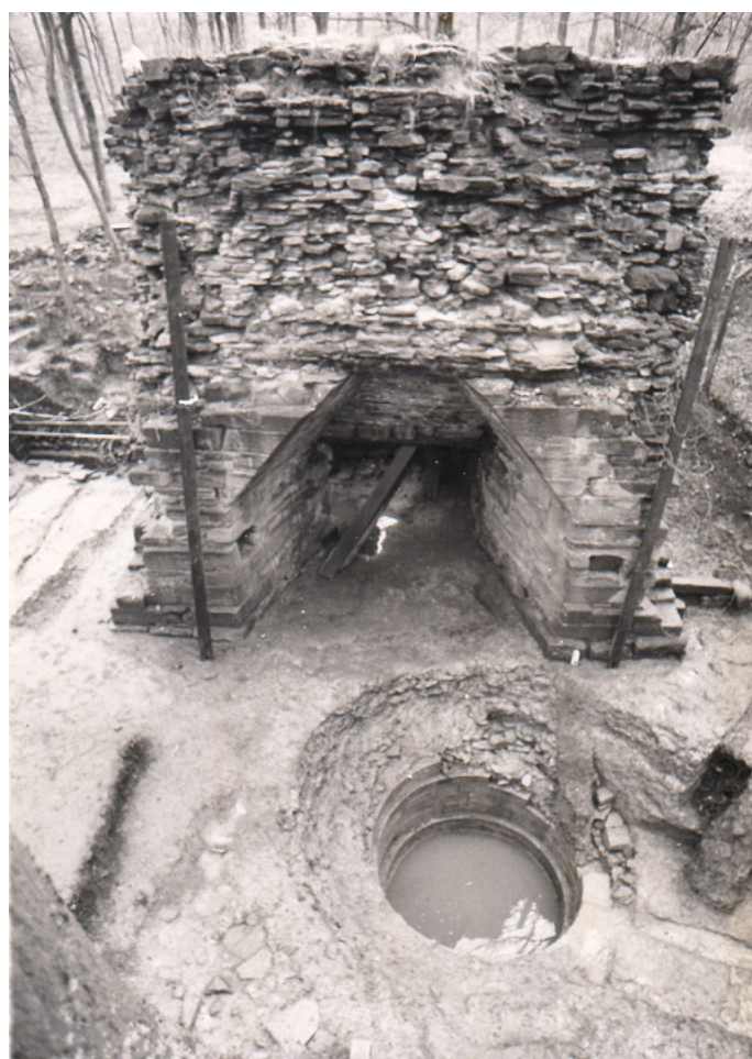
Rockley blast furnace c. 1700 during excavations in the 1980s by David Crossley (note casting pit in foreground). Rockley is located close to junct 36 M1 north of Sheffield.
